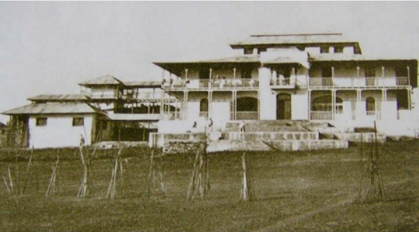
Figure 6. Taytu Hotel - Southern Façade. Ca. 1910.
